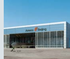
Ameco A380 Hangar Peking, China
